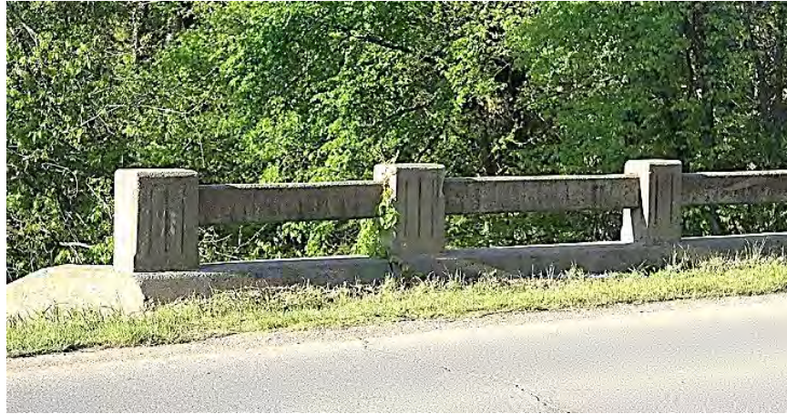
TL 2 Option: Natchez Trace Concrete Bridge Railing
