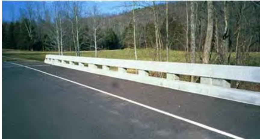
TL 2 Option 1: Natchez Trace Concrete Bridge Railing
