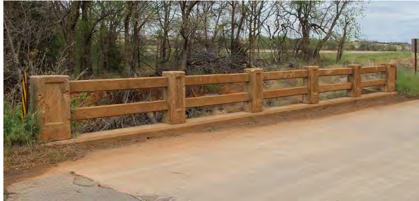
TL 2 Option 1: Natchez Trace Concrete Bridge Railing
