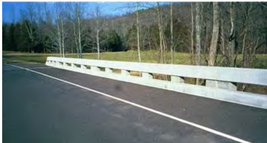
TL 2 Option: Natchez Trace Concrete Bridge Railing
