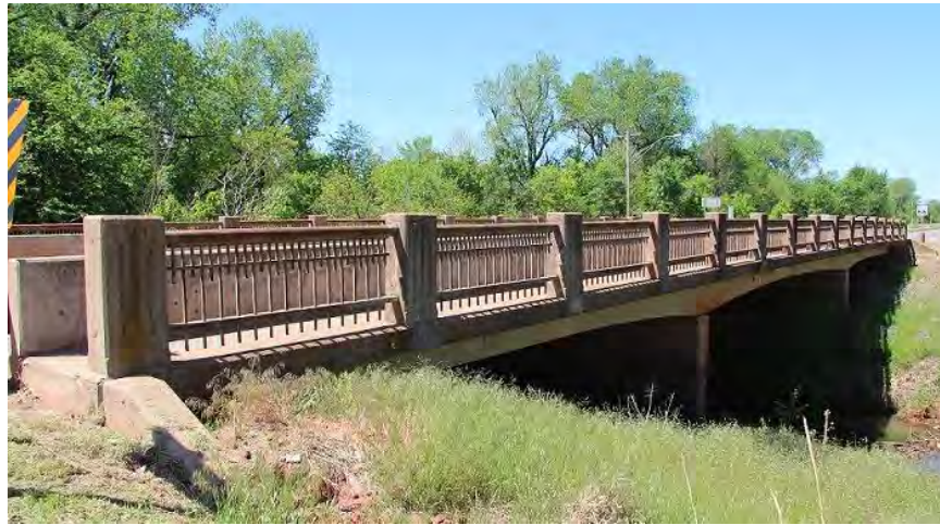
TL 2 Option: Washington, D.C. Historic Bridge Rail Retrofit (Curb Mount)
