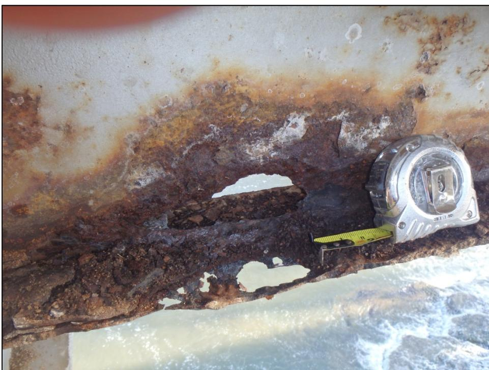
Figure 4 – Corrosion Holes in Stringer
