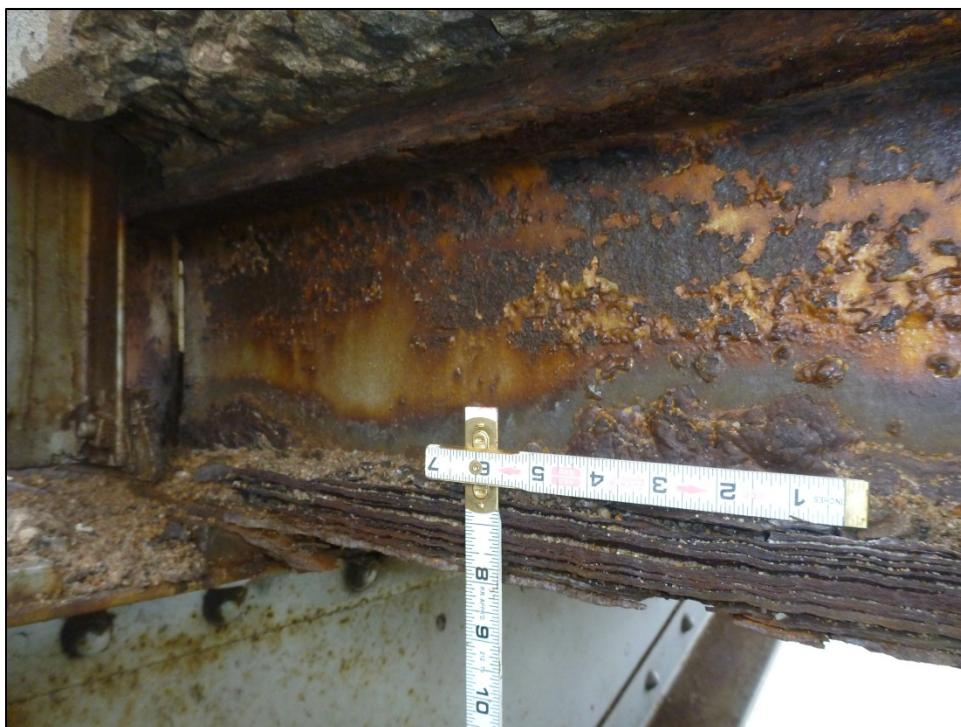
Figure 5 – Corrosion and Impacted Rust on Stringer Flanges
