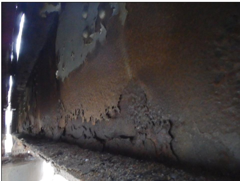
Figure 6 – Section Loss at Web of Floorbeam
