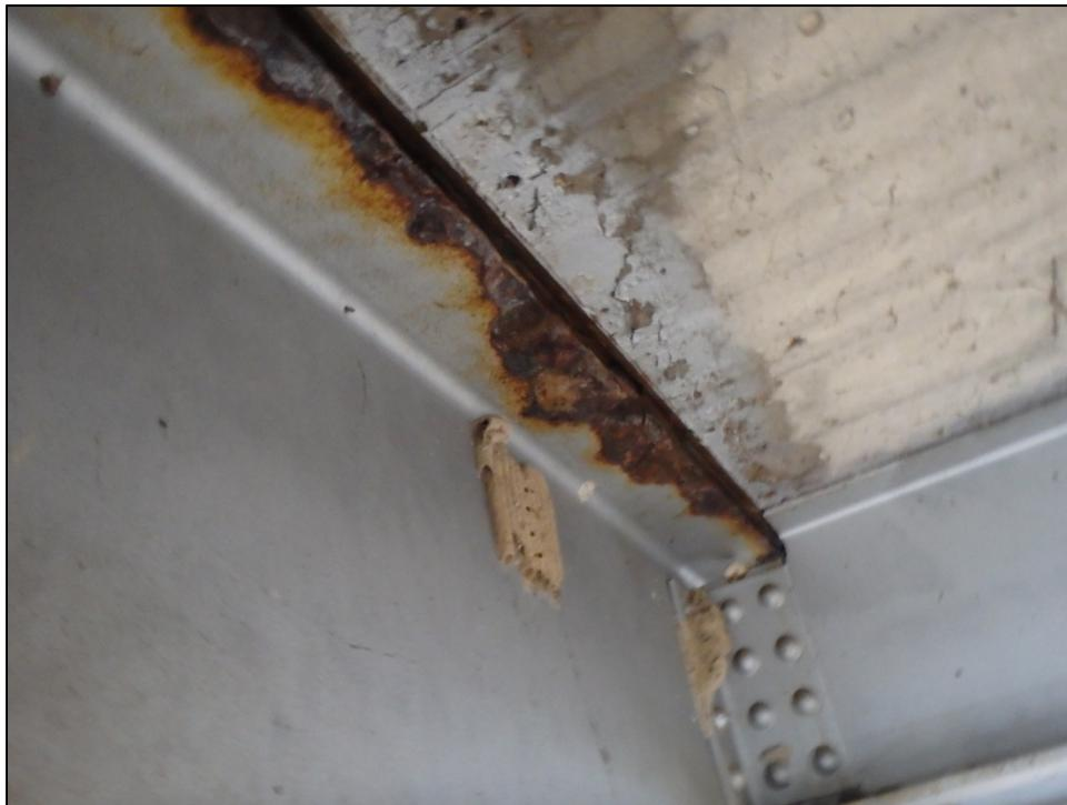
**Figure 7 – Corrosion and Impacted Rust at Floorbeam Top Flange**
