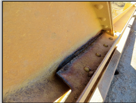
Figure 22. Corrosion at Welded Connection of Rail to Truss Member
