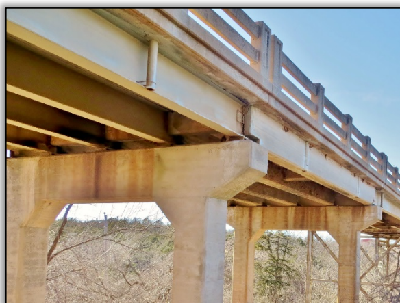
Figure 44. Steel Beam Span and Concrete Encased Steel Beam Span
