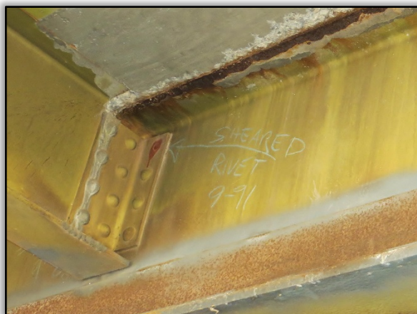
Figure 28. Sheared Rivet at Stringer-Floor Beam Connection
