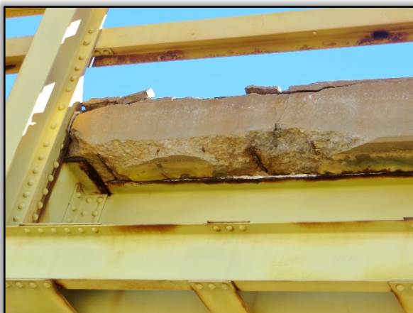
Figure 13. Typical Overhang Spall
