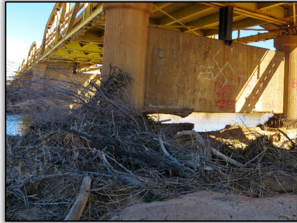
Figure 38. Debris Buildup at Pier
