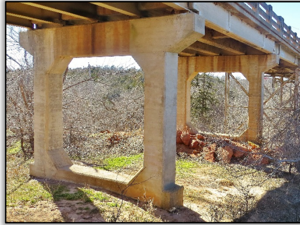
Figure 49. Concrete Piers at East End of Bridge
