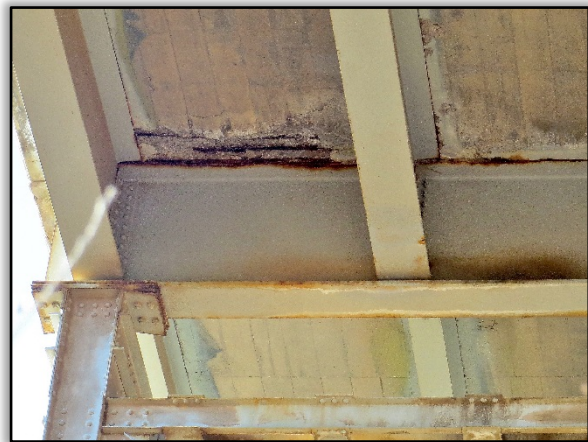
Figure 41. Soffit Spall Near Joint at Pier Beam
