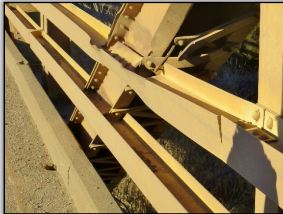
Figure 36. Collision Damage to Metal Rail
