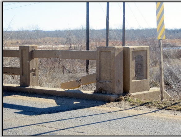
Figure 34. Failure of Concrete Rail at South End of Bridge (Span 1)
