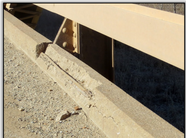
Figure 14. Typical Curb Spall
