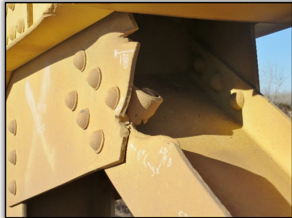
Figure 19. Torn Flange and Gusset Plate at West Truss, Span 31
