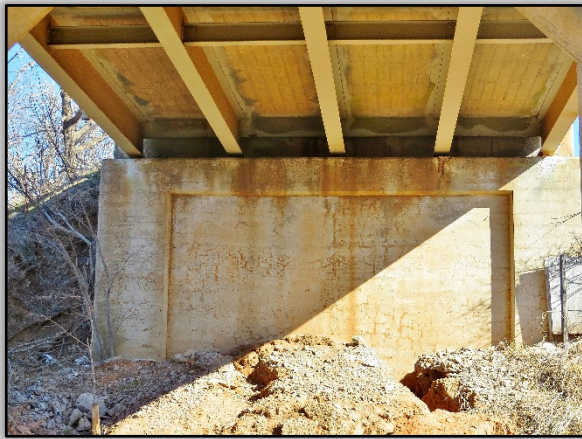
Figure 50. Map Cracking on East Abutment Face
