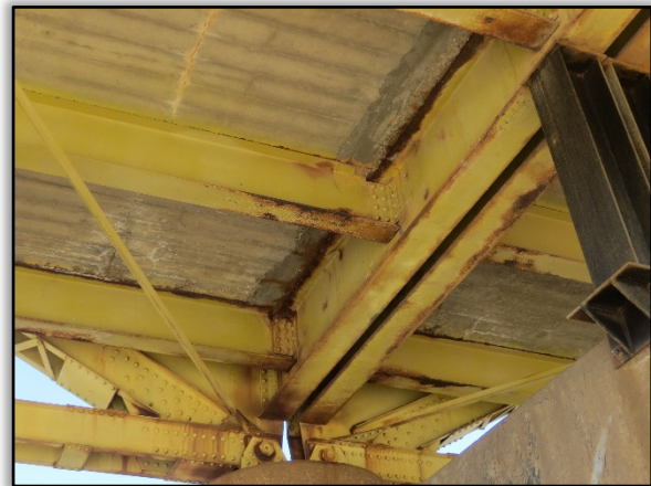
Figure 27. Corrosion of Stringers and Pier Beams
