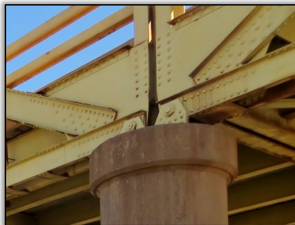
Figure 25. Outboard Truss End at Pinned Bearing
