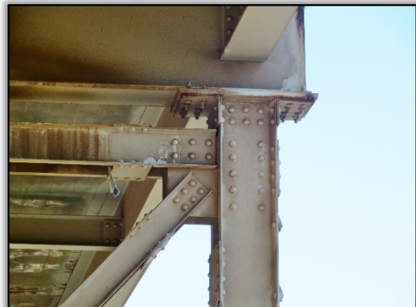
Figure 43. Connection of Floor Beam to Steel Bent
