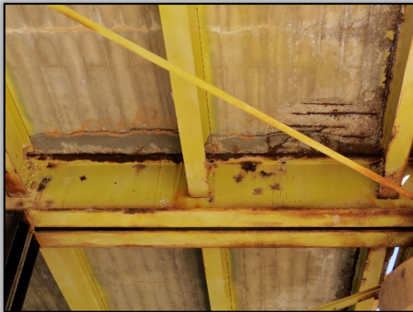
Figure 11. Spalls with Exposed Rebar and Asphalt Fill at Expansion Joint under Deck
