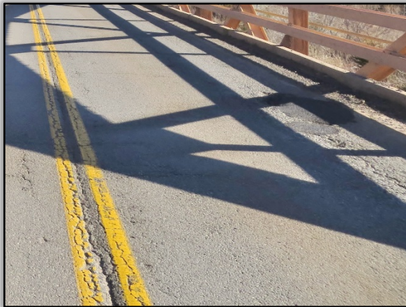
Figure 9. Typical Longitudinal Cracking in Asphalt Overlay
