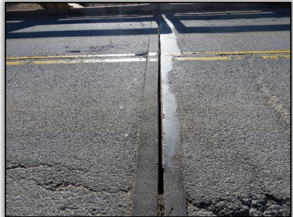
Figure 10. Typical Expansion Joint
