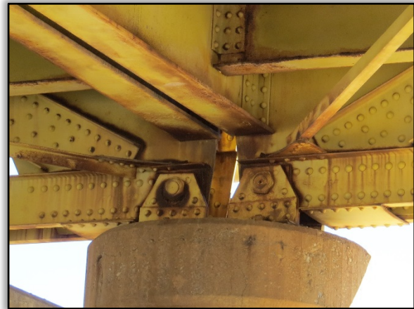
Figure 24. Deterioration of Pinned Bearing Assembly and Truss Lower Chord at Expansion Joint Between Trusses
