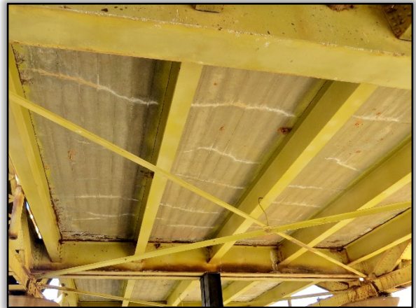
Figure 12. Transverse Cracking in Soffit
