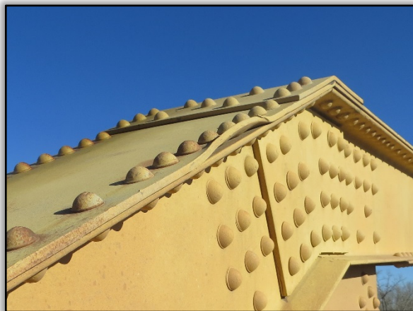
Figure 16. Typical Truss Upper Chord Collision Damage
