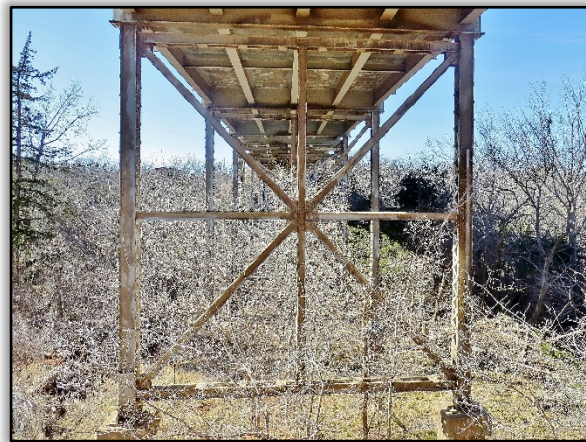
Figure 47. Steel Bent with Midpoint Bracing and Vertical Stiffeners
