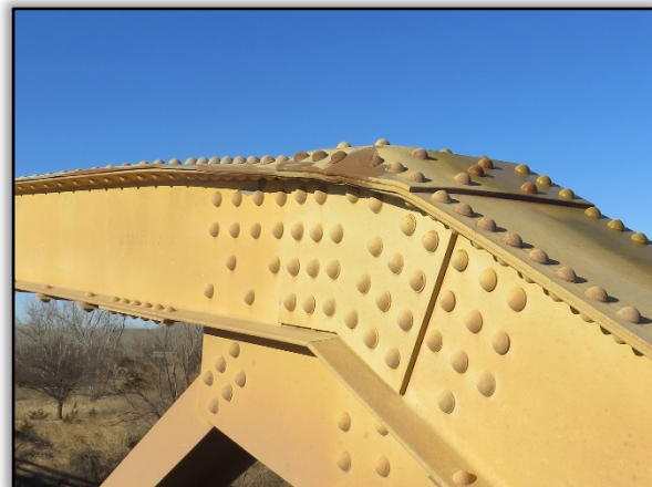
Figure 17. Gusset Plate Bowed Up and Corroded at West Truss, Span 30
