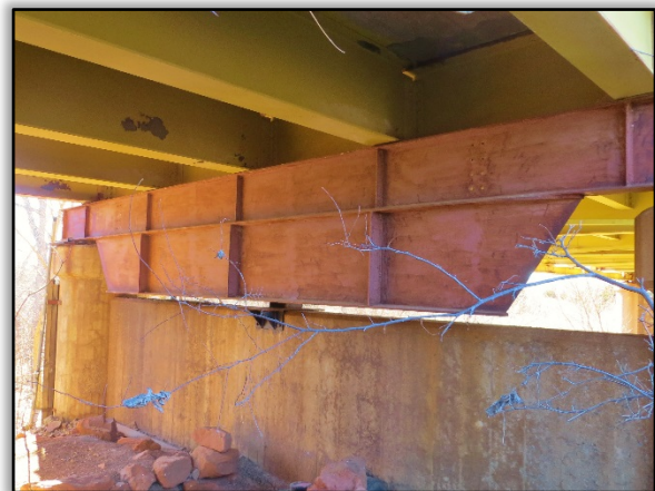
Figure 33. Supplemental Pier Beam
