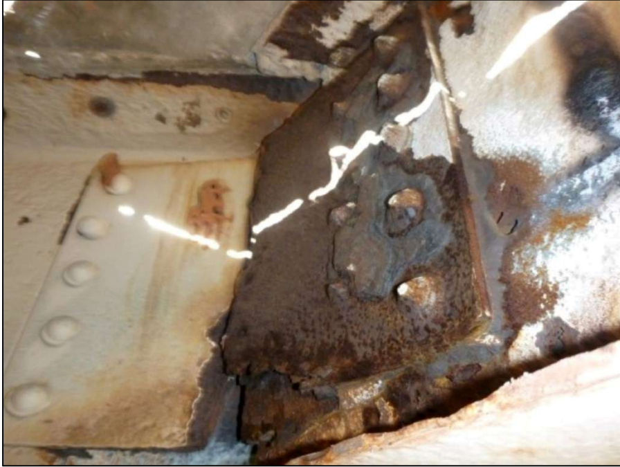
Span 2, Stringer 1 connection to Floor Beam 0, 100 percent section loss
