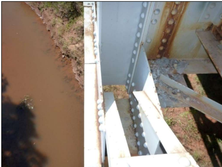
South Truss, L2 gusset plates
