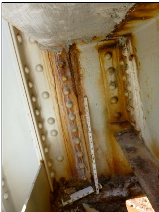
typical floor beam to truss vertical connection
