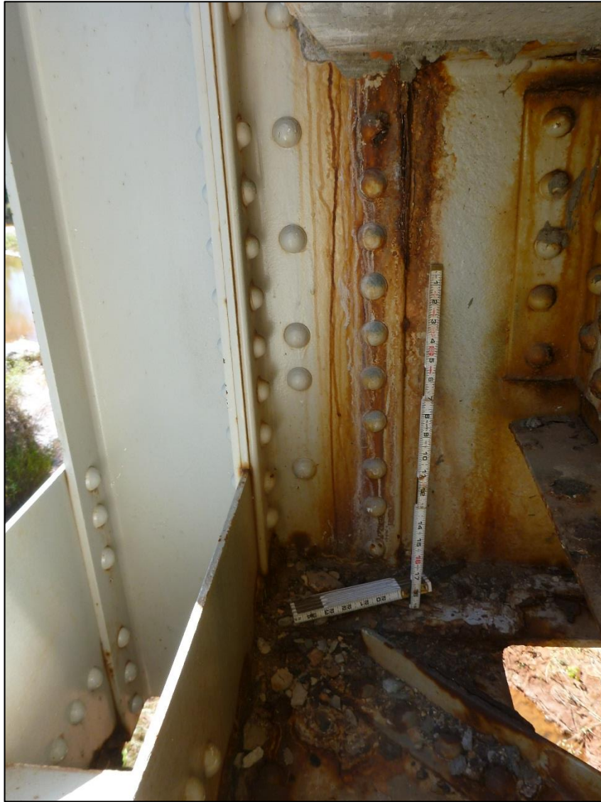
Figure 16: Typical corrosion and pack rust at floor beam to truss connection
