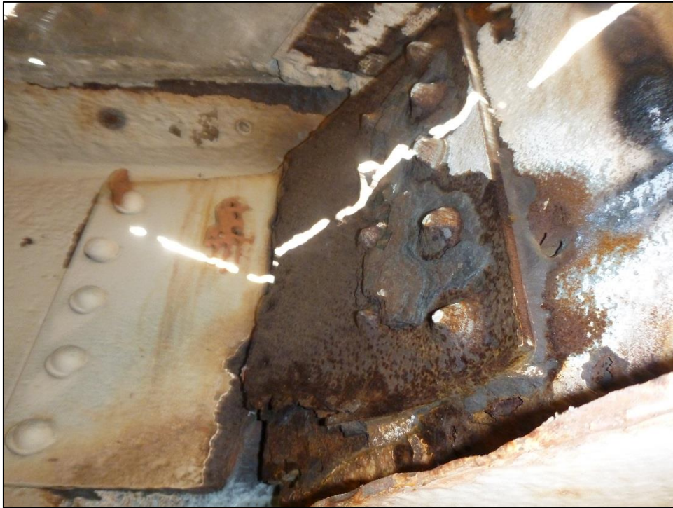
Figure 14: Span 2, Stringer 1 connection to Floor Beam 0, south side connection
