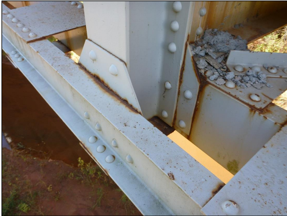
Figure 17: Span 2, North Truss, Panel Point L1 (typical of Panel Points L1 and L4 on both trusses)
