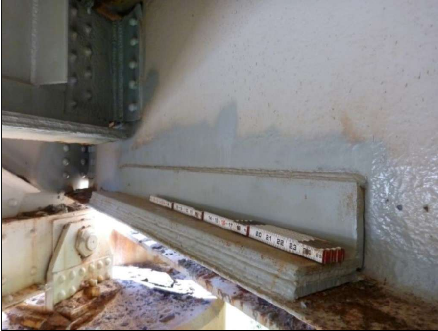
Span 2, Floor Beam 0, welded plate repair
