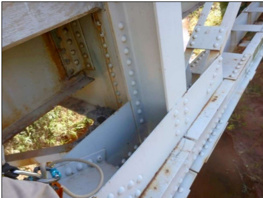
North Truss, L3 gusset plate
