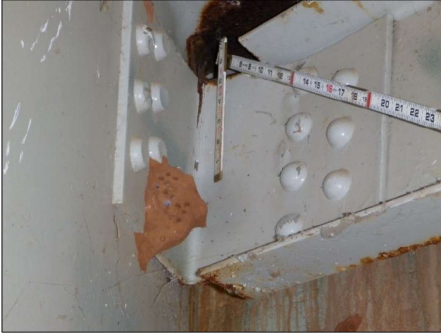
Span 1, Bay 4 diaphragm connection at Pier 1, 2-in long crack in connection angle
