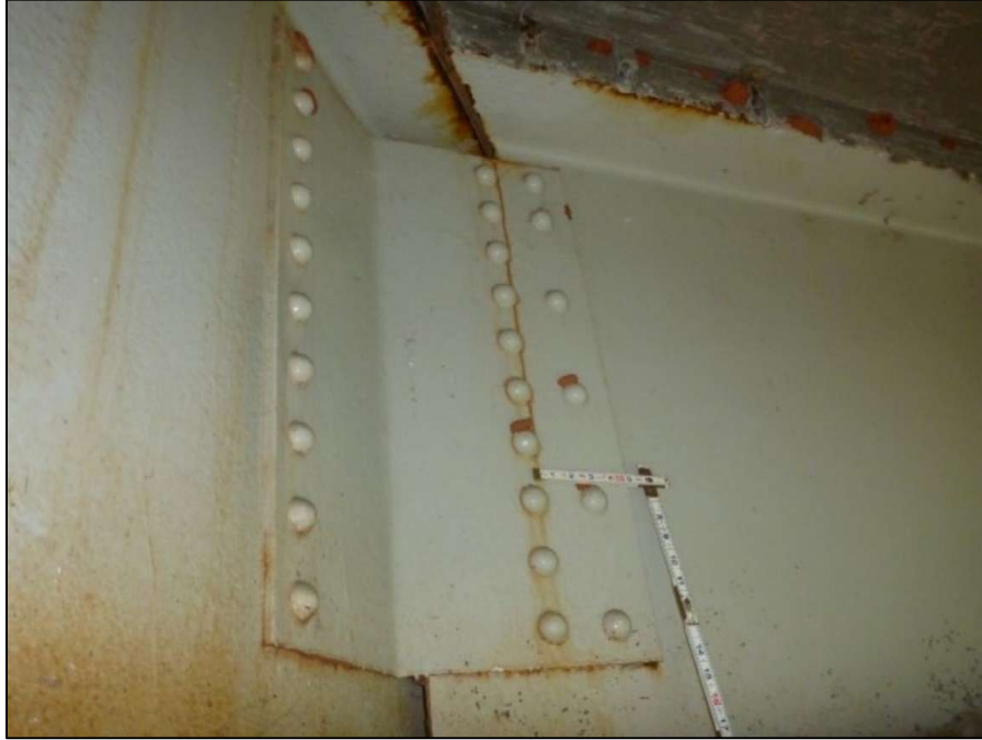
Typical stringer to pier beam connection
