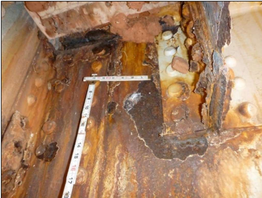
South Truss, Floor Beam 5 connection, 5/16-in deep pitting adjacent to Stringer 1
