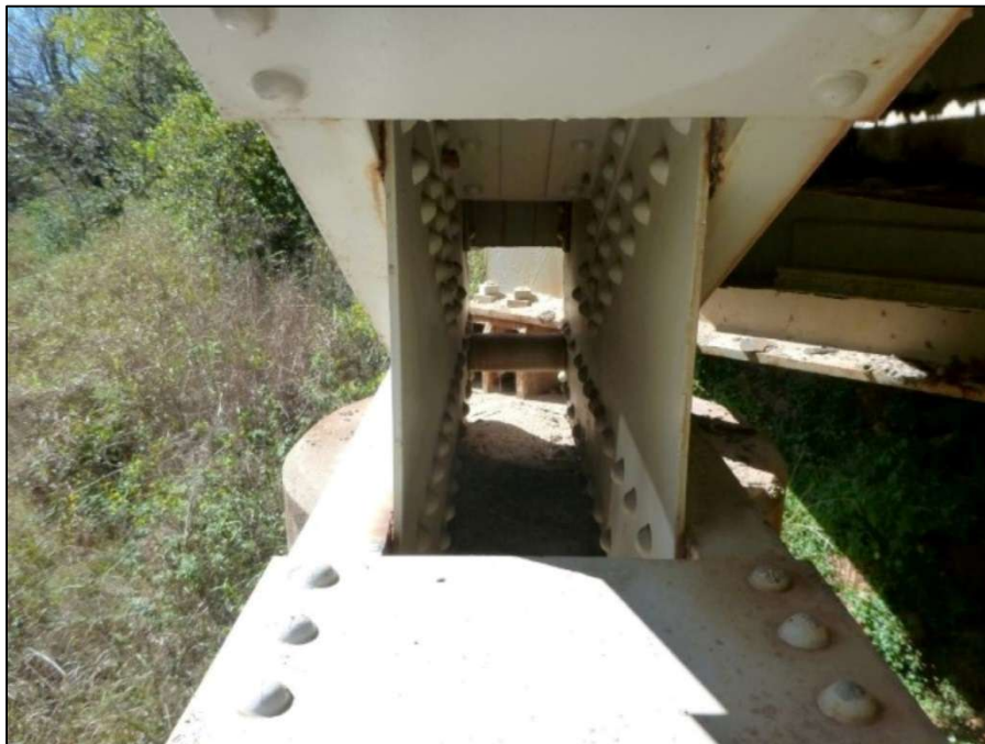
South Truss, L0 gusset plates, 1/8-in pack rust
