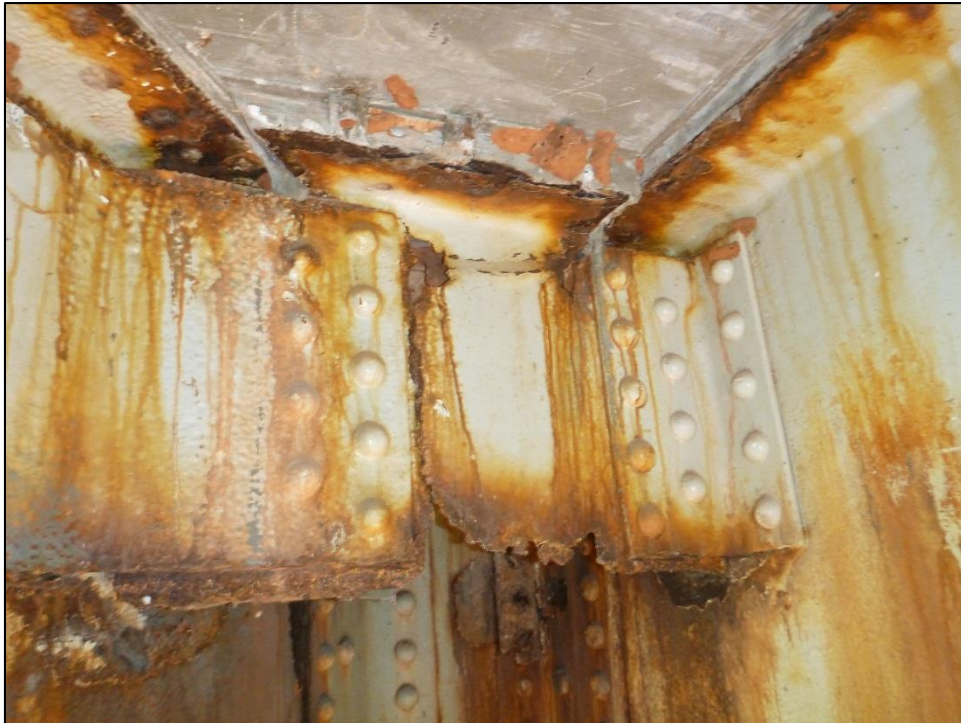
Figure 15: Span 2, Stringer 1 between Floorbeams 5 and 6, 100 percent section loss
