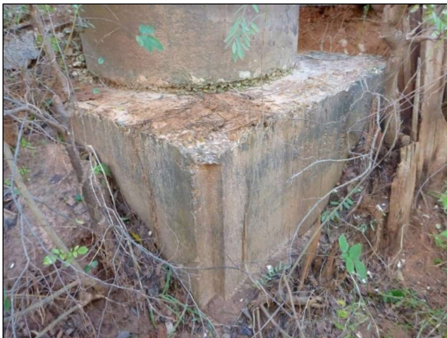
Pier 2, North Footing, 27-in high exposure
