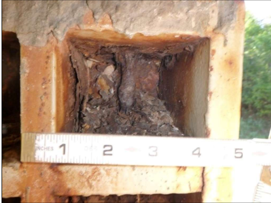
Pier Beam, South Bearing, Section loss to west anchor bolt
