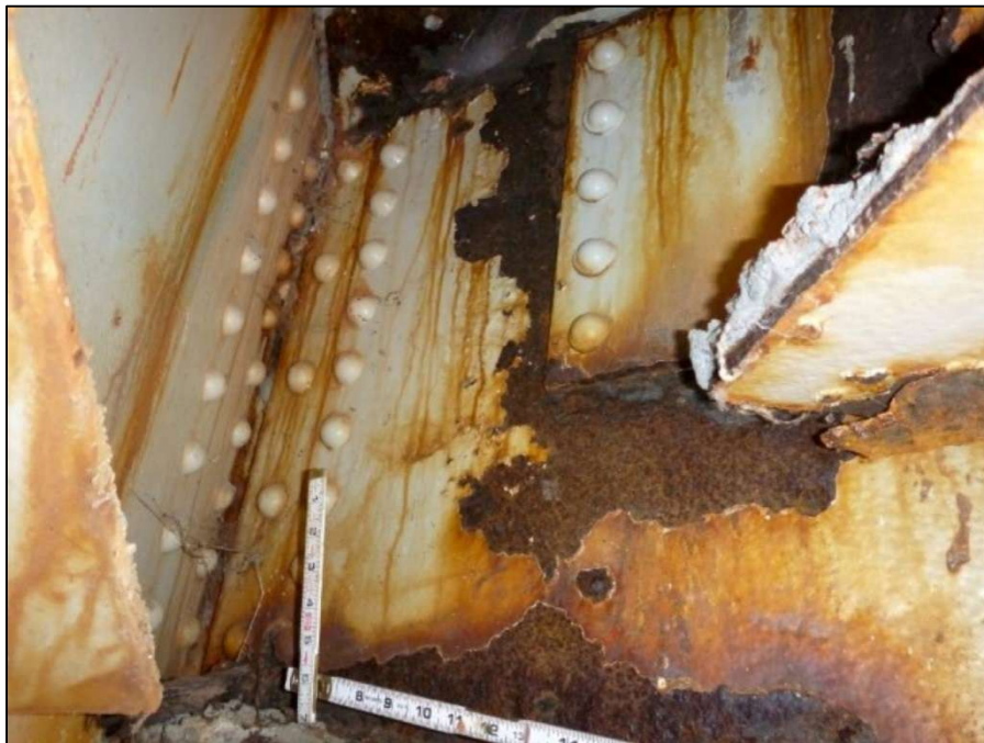
Span 2, Floor Beam 6 adjacent to stringer 5, 1/4-in D pitting
