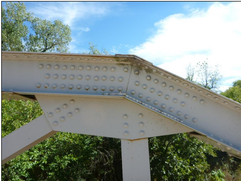
Figure 20: Span 2, South Truss, Panel Point U2 (conditions typical of upper panel points at both trusses)
