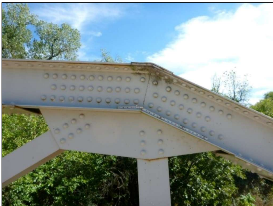
North Truss, U1 gusset plate
