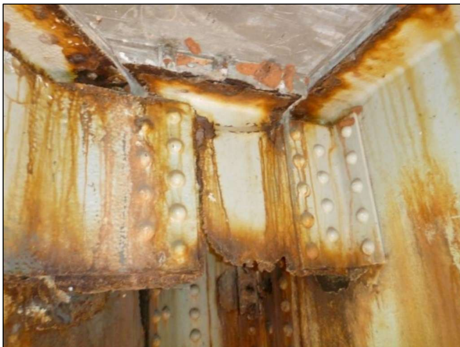
Span 2, Stringer 1 between Floor Beam 5 and 6, 100 percent section loss
