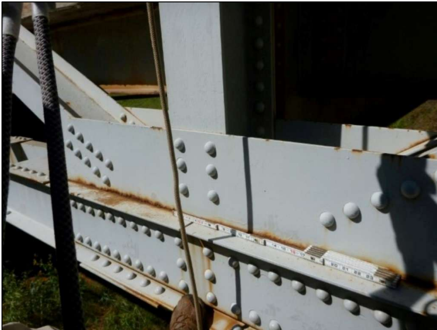
South Truss, L2, minor surface corrosion.
