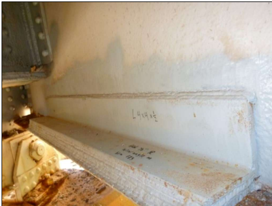
Span 2, Floor Beam 0, welded plate repair
