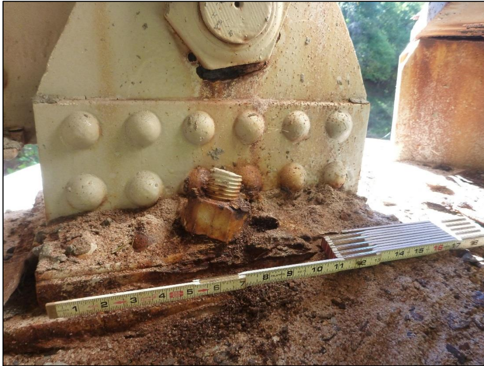
Figure 21: Span 2, North Truss, bearing at L0 (west end), anchor bolt bent to the west due to slot exceeding limits of expansion
