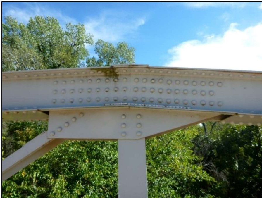
South Truss, U2 gusset plate
