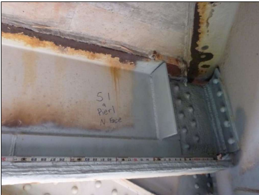
Span 2, Stringer 1 connection to Floor Beam 0, welded plate repair
