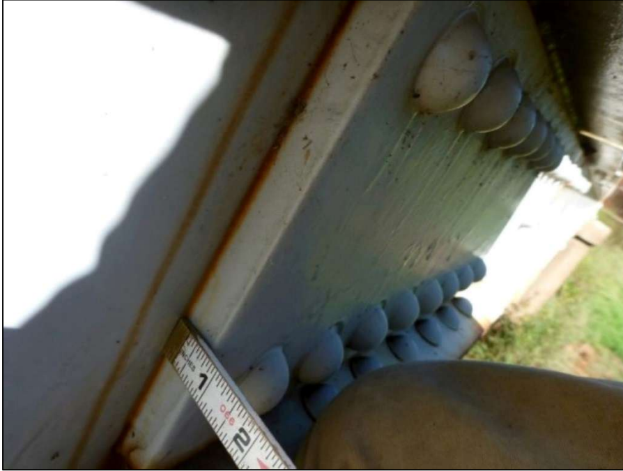
South Truss,, typical lower chord web splice plate surface corrosion
