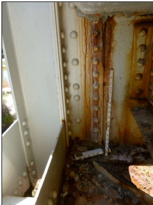
typical floor beam to truss vertical connection
