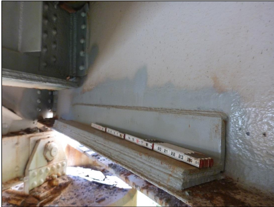
Figure 12: Span 2 (main span), Floor Beam 0, strengthening angle & plate
