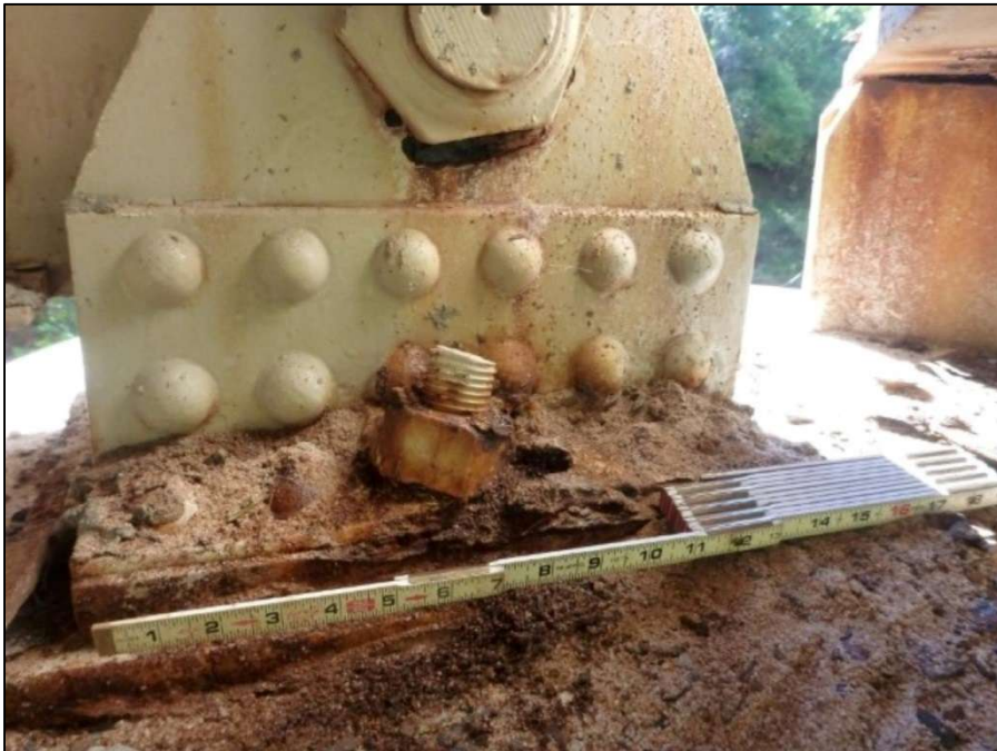
South Truss, L0 bearing, bent to the west
