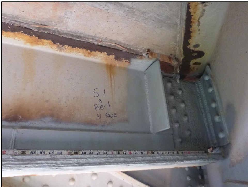
Figure 13: Span 2 (main span), Stringer 1 at Floor Beam 0, previous repair
