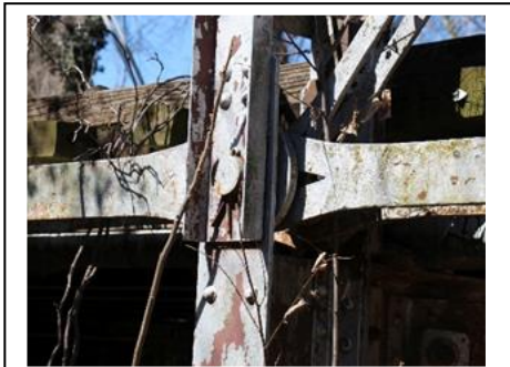
Eyebars – bottom chord.
