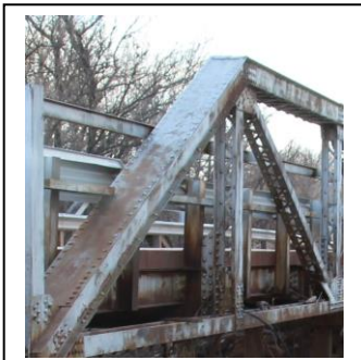
Built up - top chord, verticals and diagonals.
