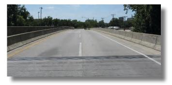
The fourth bridge is located about 500 feet east of the twin bridges over the Caney River. This bridge is a three 50 foot span I-Beam bridge carrying four lanes of traffic. The NBI Number is 21083. The bridge is rated as Not Deficient with a Sufficiency Rating of 68.6.
