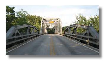
This bridge is rated as Functionally Obsolete due to the substandard width and vertical clearance of the bridge. The existing roadway width is 24 feet and the existing vertical clearance is 15 feet 6 inches. The current standards are 32 feet and 16 feet respectively for a new bridge. The bridge is also rated as Structurally Deficient because of the bridge superstructure.
