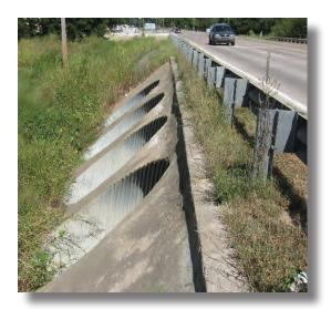
There are four bridges on Tuxedo Boulevard within the study limits. The first bridge is about 3,700 feet east of Cherokee Avenue. This bridge is a culvert with 4-8.5' diameter corrugated galvanized steel pipe (CGSP). The NBI Number is 20708. The bridge is rated as Not Deficient with a Sufficiency Rating of 78.9.
