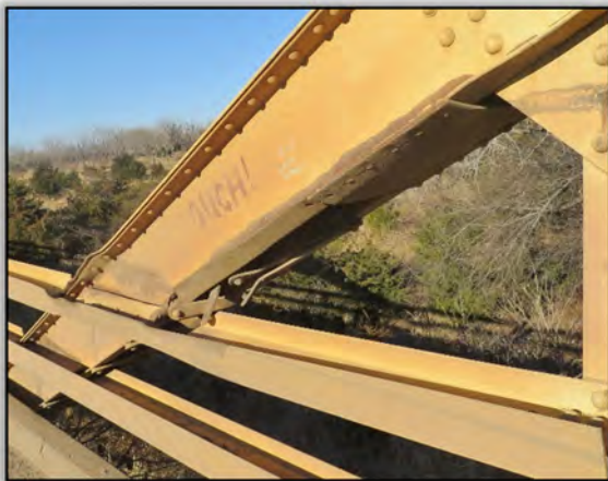
Figure 20. Bent Flanges and Rail, Disconnected Lacing, Sheared Rivets at West Truss, Span 31
