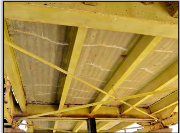
Figure 12. Transverse Cracking in Soffit
