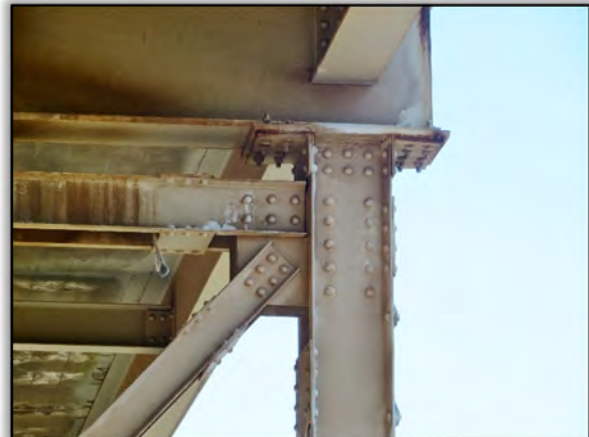
Figure 43. Connection of Floor Beam to Steel Bent
