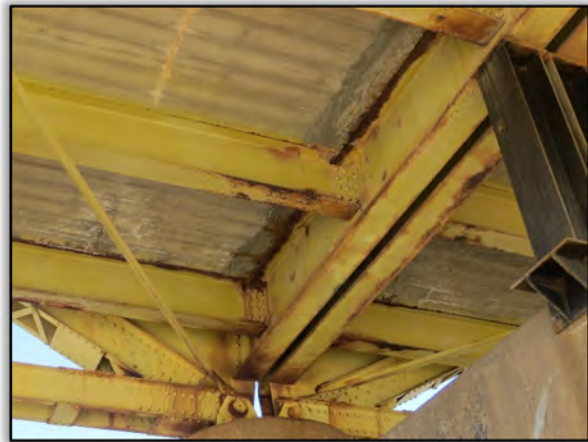
Figure 27. Corrosion of Stringers and Pier Beams
