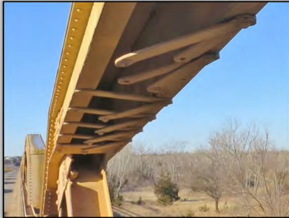
Figure 18. Disconnected Lacing with Sheared Rivets at West Truss, Span 31
