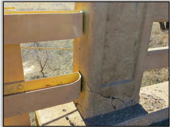
Figure 35. Damage to Concrete Rail Due to Impact from Metal Rail
