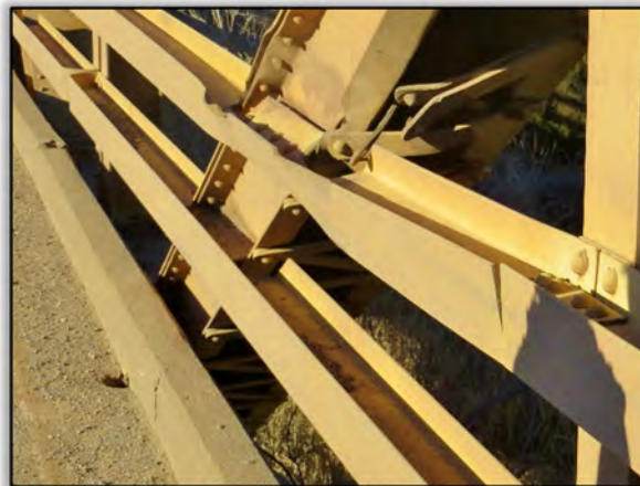
Figure 36. Collision Damage to Metal Rail
