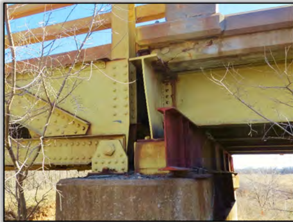
Figure 32. Pier Beam Rotation at South End Span and Supplemental Pier Beam
