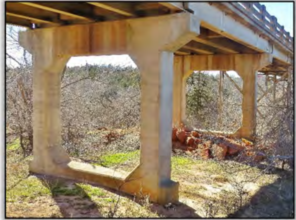
Figure 49. Concrete Piers at East End of Bridge
