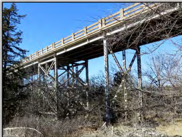
Figure 46. Bridge Elevation Showing a Typical Steel Tower (Left) and Steel Bent (Right)
