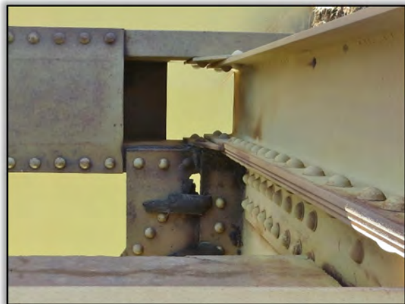
Figure 29. Corrosion Hole in Floor System Bracing Gusset Plate at Connection to Truss
