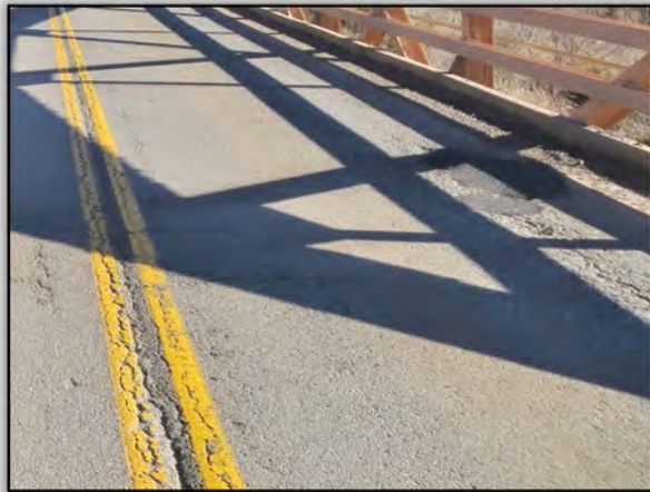
Figure 9. Typical Longitudinal Cracking in Asphalt Overlay
