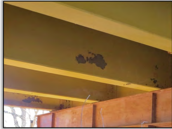
Figure 31. Corrosion near Beam Ends in North End Span
