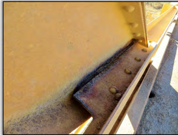
Figure 22. Corrosion at Welded Connection of Rail to Truss Member
