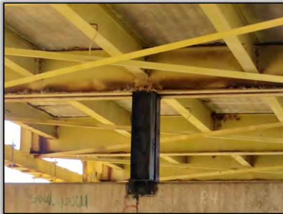
Figure 26. Typical Stiff Leg between Steel Pier Beam and Concrete Pier Wall
