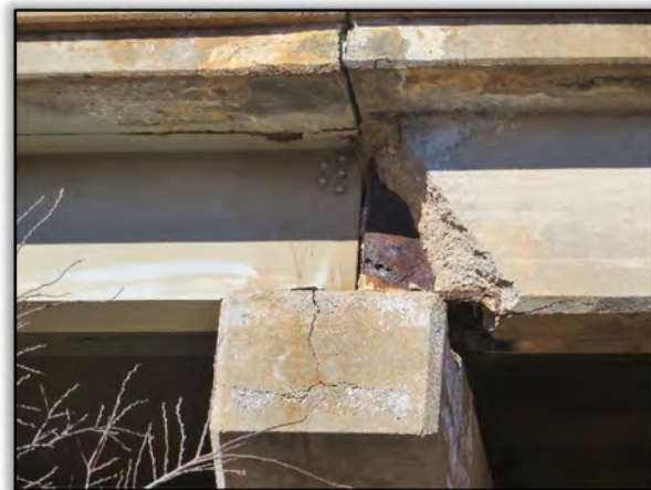
Figure 45. Spalled Concrete Encasement Revealing Corroded Steel Beam End
