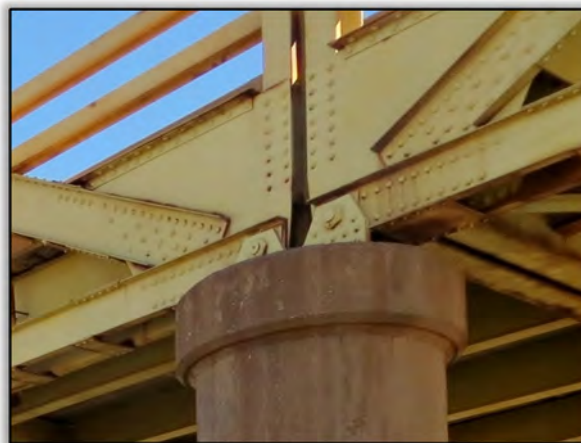
Figure 25. Outboard Truss End at Pinned Bearing
