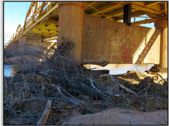
Figure 38. Debris Buildup at Pier
