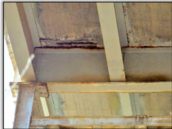
Figure 41. Soffit Spall Near Joint at Pier Beam
