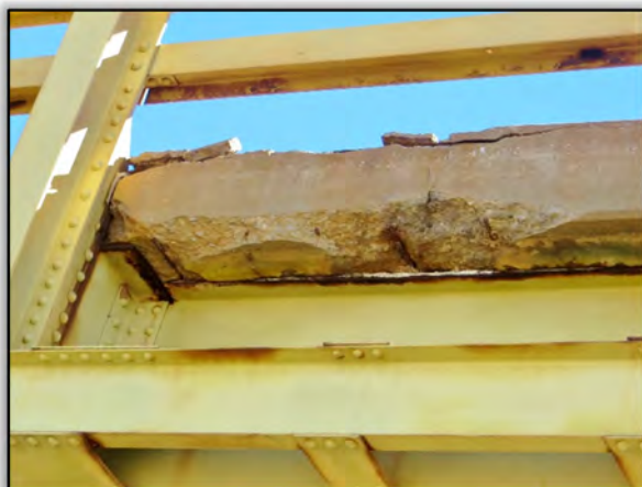
Figure 13. Typical Overhang Spall
