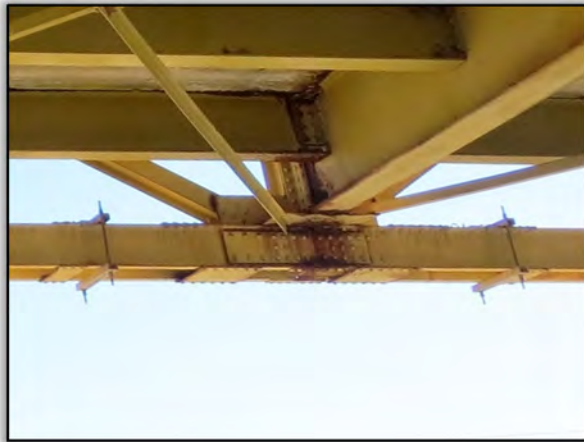
Figure 23. Corrosion at Inboard L2 Gusset Plate Beneath Deck Construction Joint
