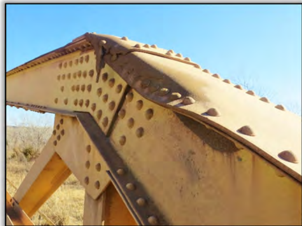
Figure 21. Bent, Torn, and Corroded Top Flange at East Truss, Span 14
