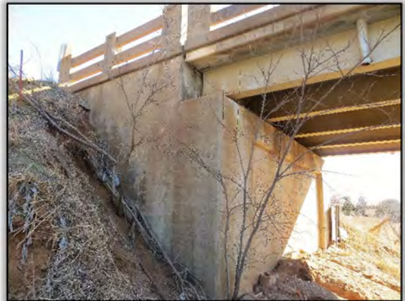
Figure 51. Map Cracking on North Wing of East Abutment
