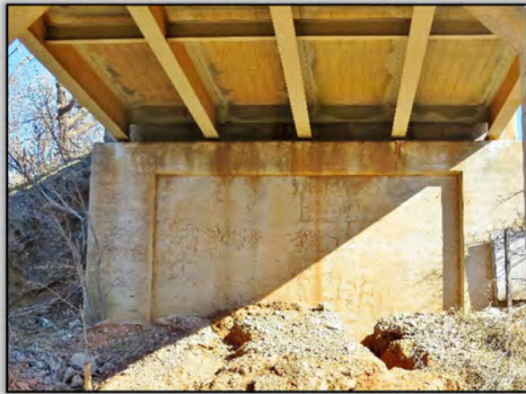
Figure 50. Map Cracking on East Abutment Face
