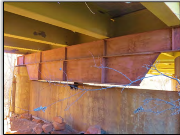
Figure 33. Supplemental Pier Beam
