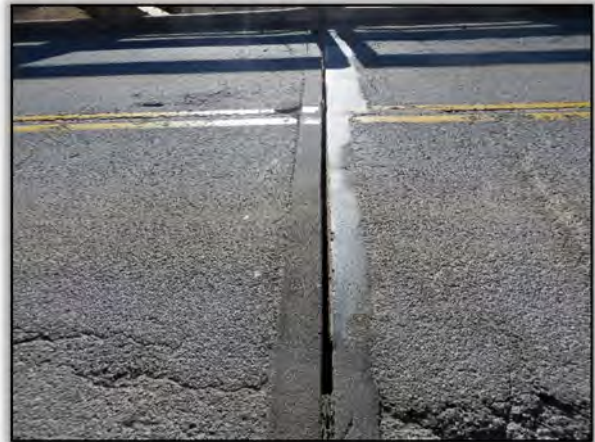
Figure 10. Typical Expansion Joint
