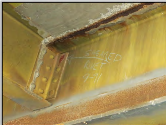
Figure 28. Sheared Rivet at Stringer-Floor Beam Connection
